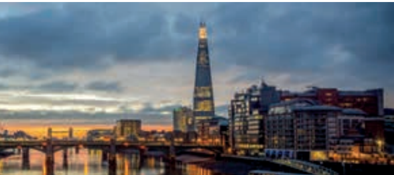
SPP project: The Shard - London
