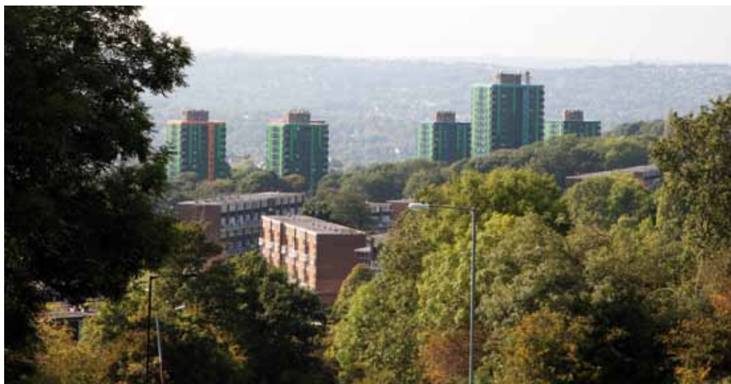
A view across Callow Mount. One of these 13-storey towers was chosen for the pilot retrofit project, and BAFSA was granted a licence by the City Council to manage the project.
