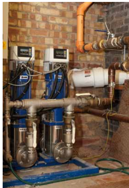
The four internal service mains in the block provided the water for the sprinkler system. Twin electric pumps supplement the service main's supply although, during installation, the mains pressure was tested and the 1.5bar reading at the top floor was in any case judged sufficient for the system.
