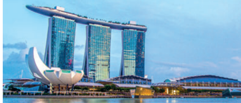
SPP project: Marina Bay Sands - Singapore
